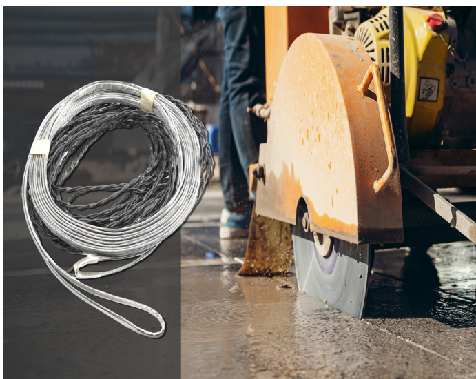
Saw Cut Loop Installation
